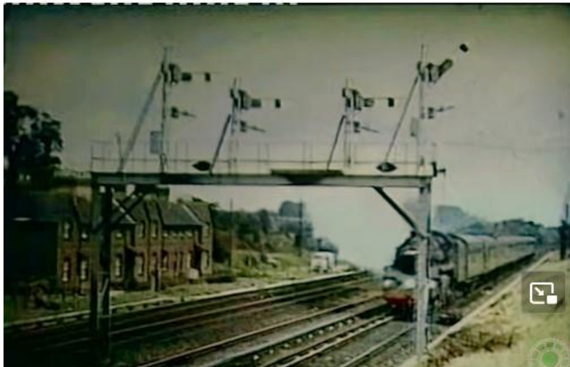
Fig 9a Cottages west of Worthing Bridge
